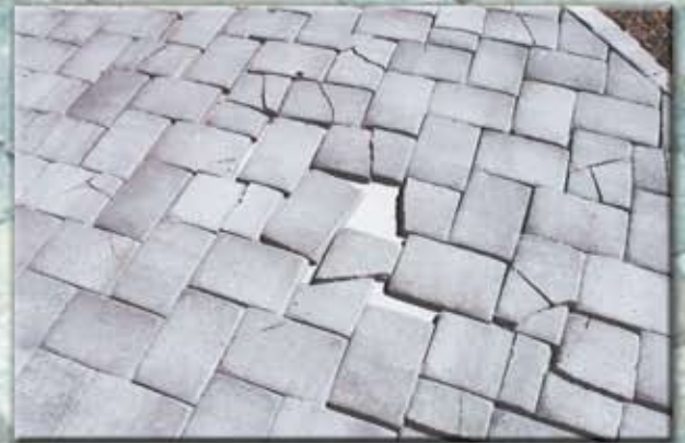
Excessive Cracking
